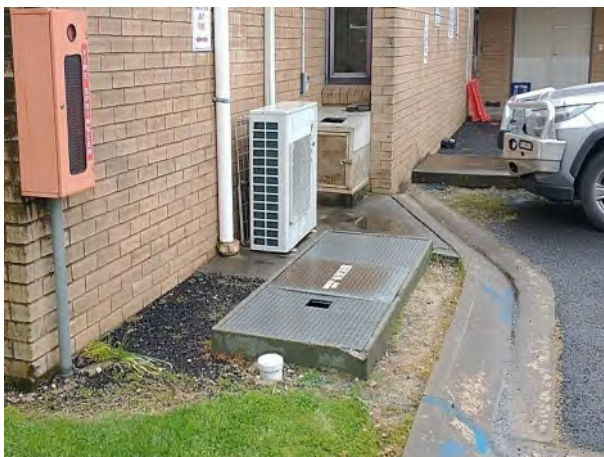
Photographs 3: Grease trap at rear of main building (west) (refer to Figure 2).
