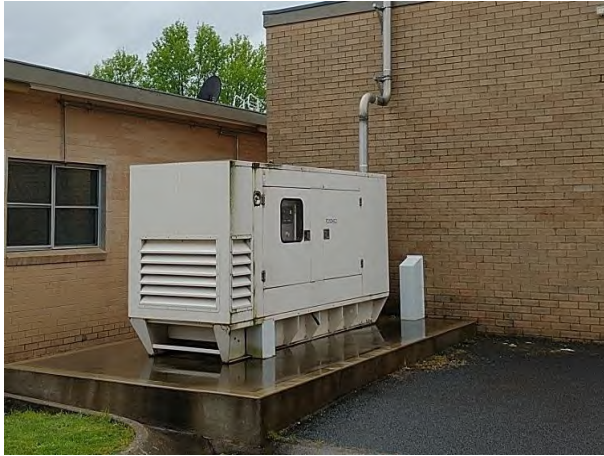
Photograph 1: Hospital back-up generator within in-built diesel tank (refer to Figure 2).
